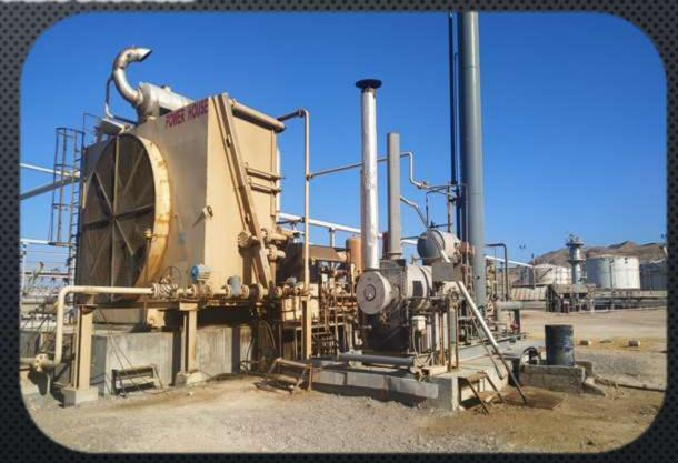
RENTAL OF DRESSER-RAND GAS COMPRESSOR FOR GAS LIFT DELIVERING 5 MMSCFD GAS FROM 37 PSI SUCTION PRESSURE TO 1300 PSI DISCHARGE PRESSURE TO INCREASE CRUDE OIL PRODUCTION.
